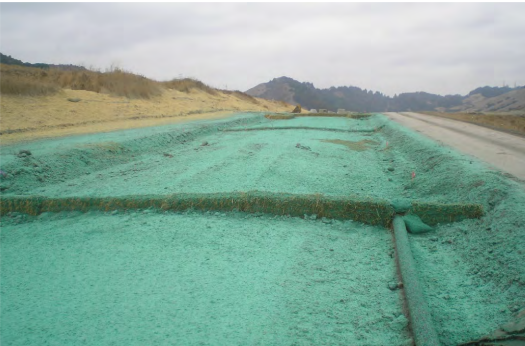
Spray on Erosion Control BMPs
