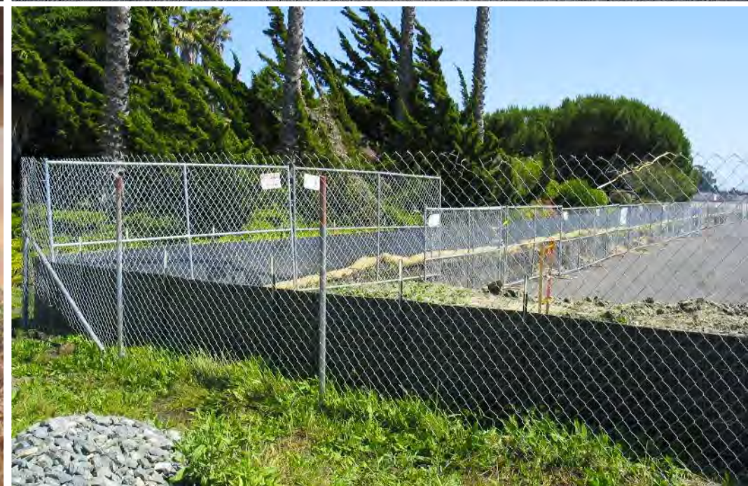
Examples of Good Silt Fence Installation
