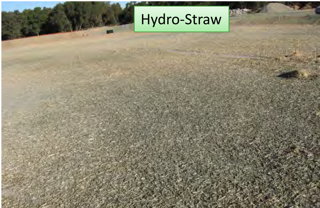
Spray on Erosion Control BMPs
