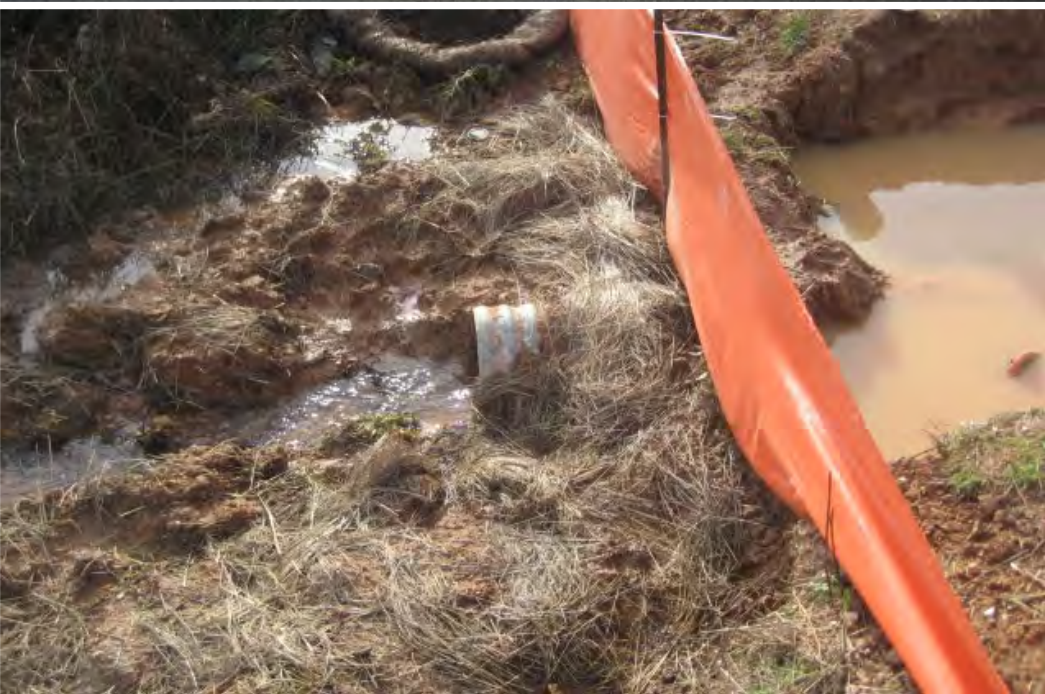
Examples of Good Silt Fence Installation
