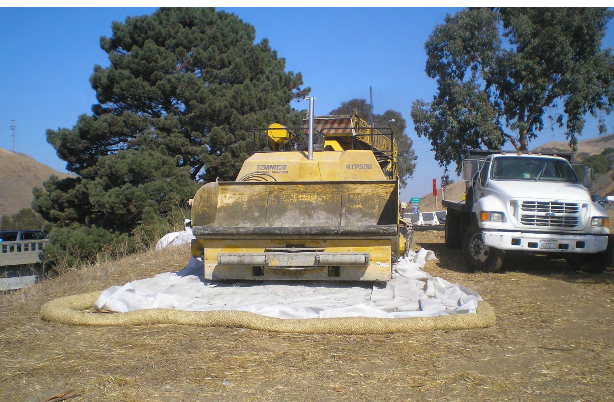
Leaking Equipment – Underline & Berm
