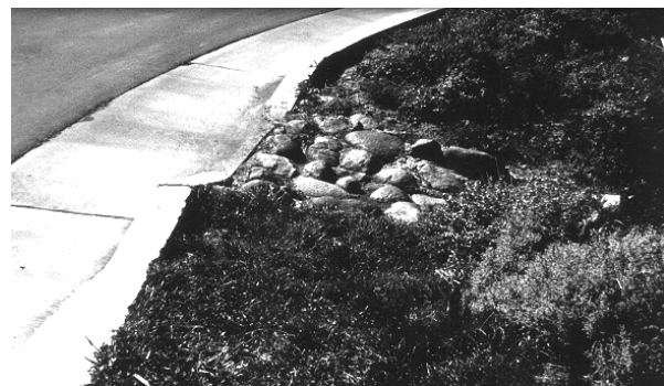
Inlet detail for urban curb/swale system
