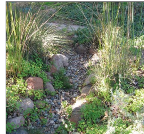
Dry creek infiltrates and conveys runoff.
